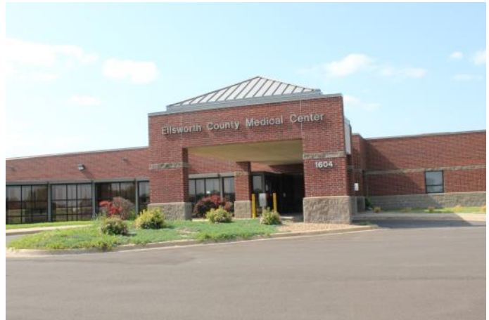
Photo 6.2: Ellsworth County Medical Center Source: Marvin Planning Consultants
